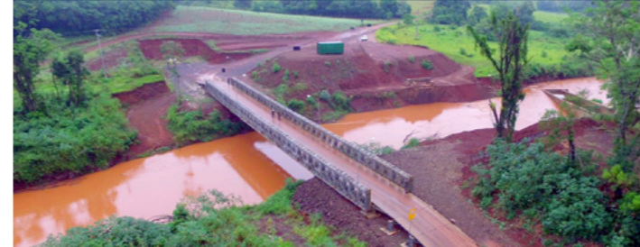
Mabey Logistic Support Bridge™, Brazil
