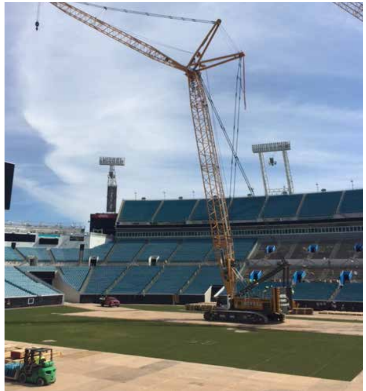
Mats protect field during stadium improvements in Florida.
