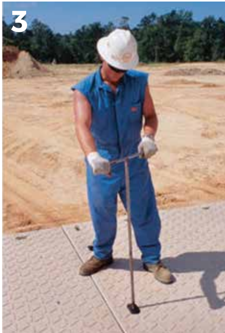
3 Pin fasteners lock mats into place to prevent separation.
