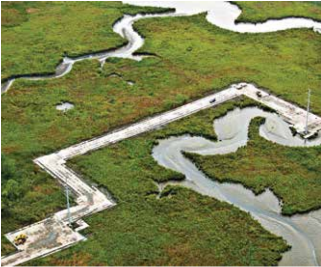
Transmission pole replacement in Maryland.
