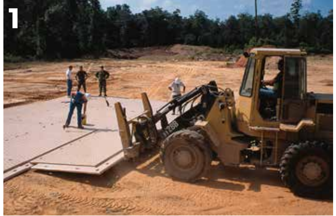
1 Mats are installed with standard site equipment.
