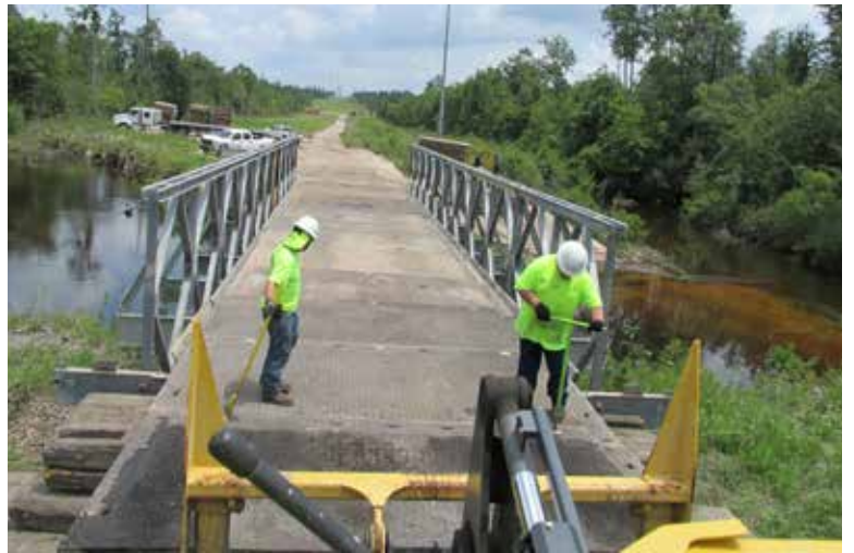
Utility project with matting over Mabey bridge in Alabama.
