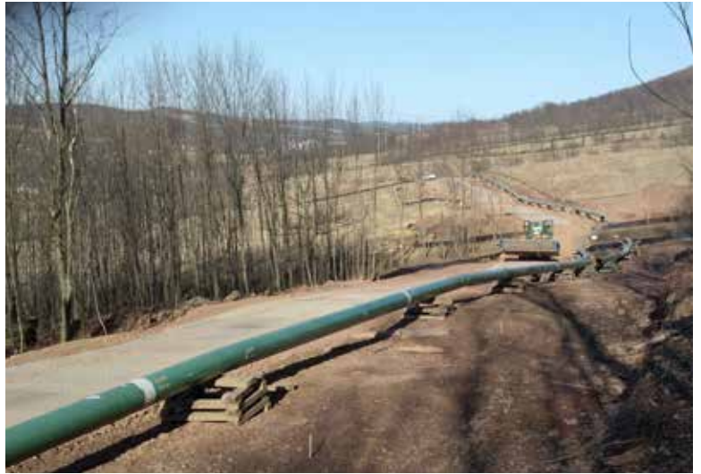
Pipeline installation in Pennsylvania.
